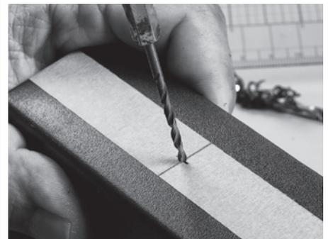
**ii.** Gradually increase the size of your drill bit until the diameter of the hole is the same as the diameter of the output cable.
